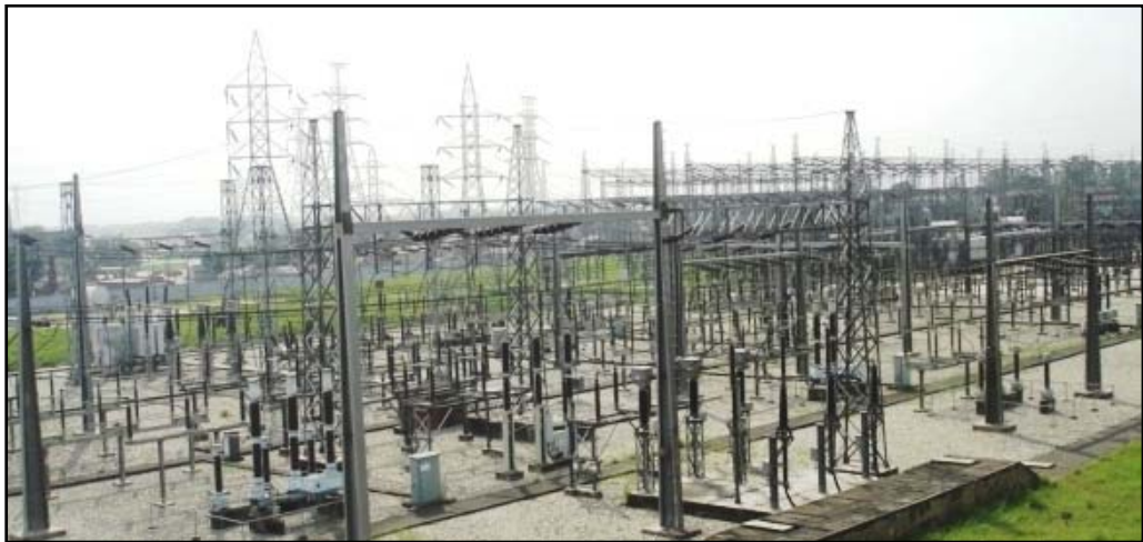
132KV & 230KV Sub-station of APSCL
