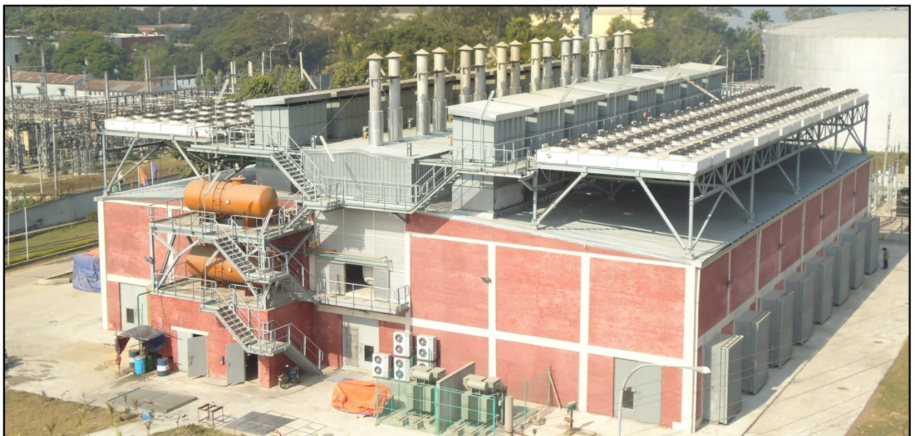
50MW Gas Engine Power Plant
