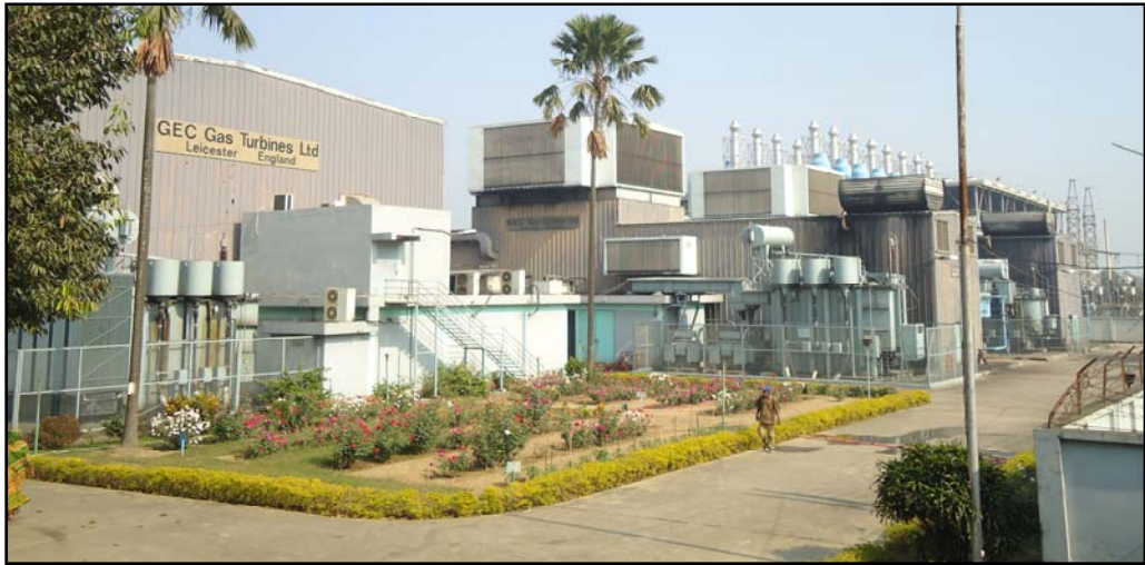
GT-1, GT-2 & ST (146 MW CCPP)
